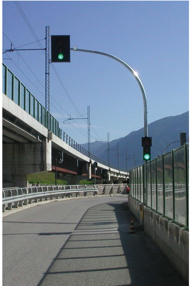
RLV radar, used on traffic light systems for speed control
