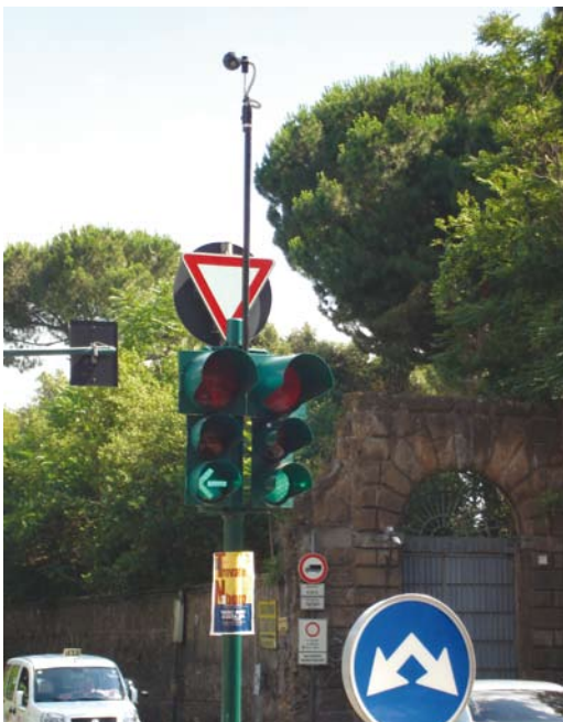
Installation on traffic light pole
